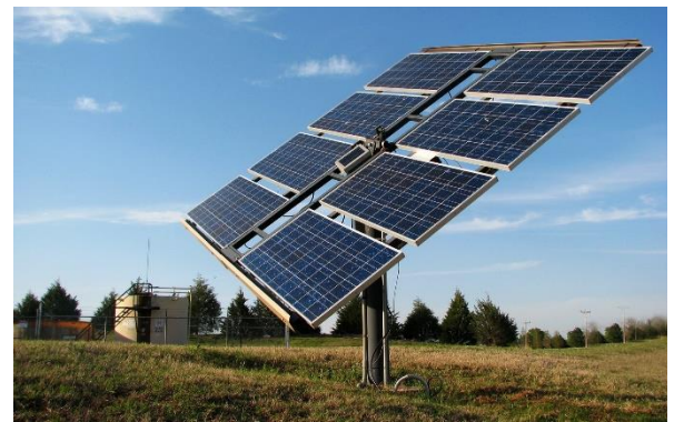
Figure 3 Example of Dual axis pole ground mount with Solar Tracking
