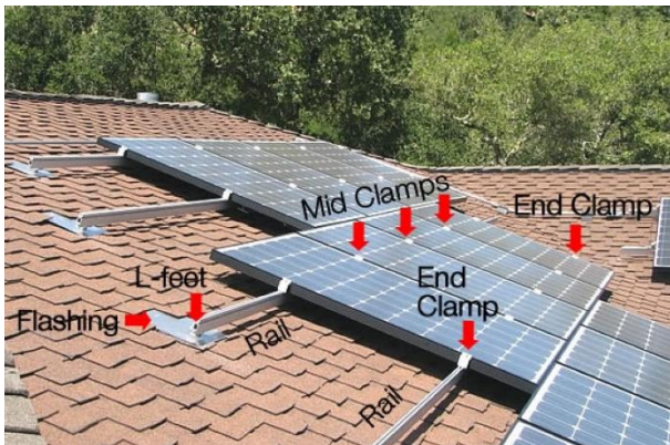
Figure 1 Example of Railed Mounting
