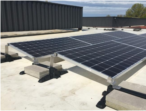
Figure 2 Example of Ballasted Roof Mounting
