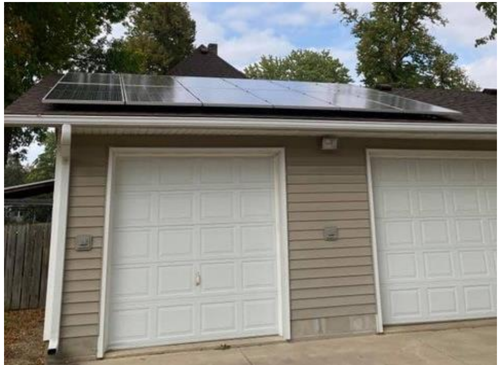
Figure 6 Example of Emily Bruce's Solar Array installed on a detached garage- 4.8 kW
