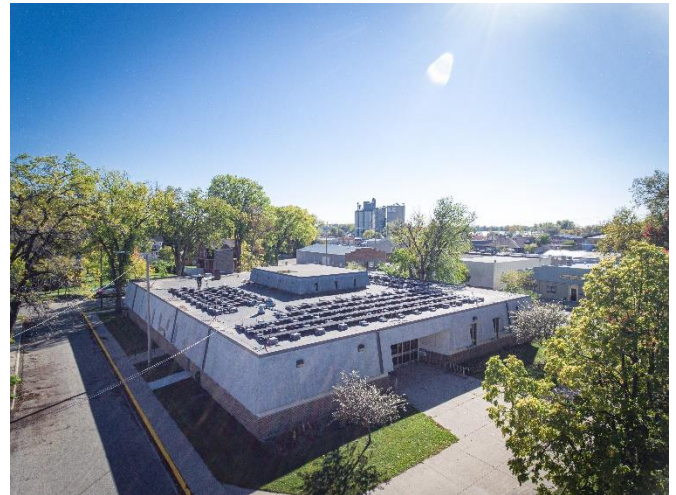
Figure 7 Solar on Morris Public Library, another ballasted roof mount.
