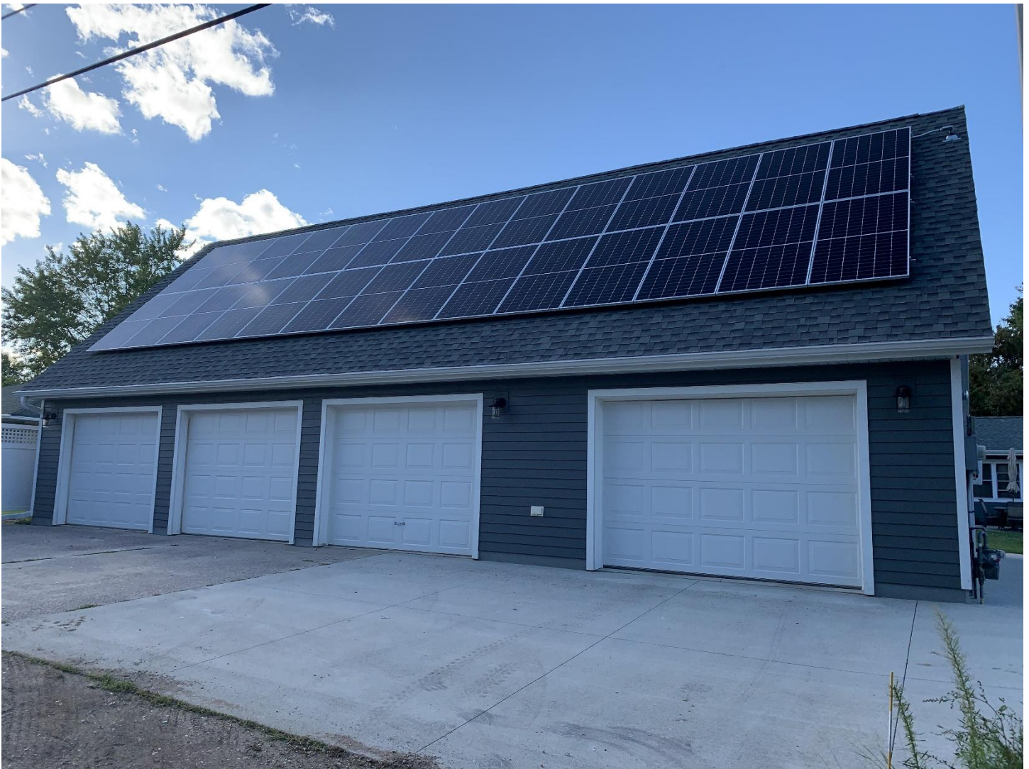
Figure 9 Bob Culbertson's finished array- 10 kW
